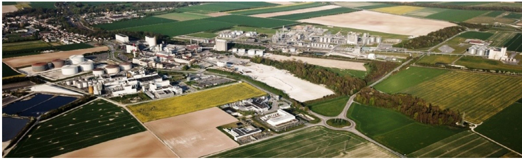
Fig. 1. Overview of the site.
